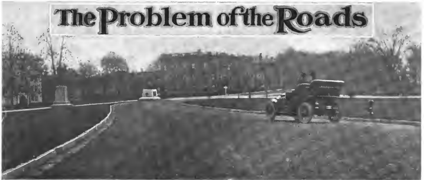
Coal Tar Treated Roadway South of the State Capitol at Hartford, and Leading Out of the Capitol Grounds.
